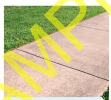
Figure 2.41 Temperature erosion causes materials such as concrete to crack. Footpaths have grooves in them to allow for their expansion during hot weather.
