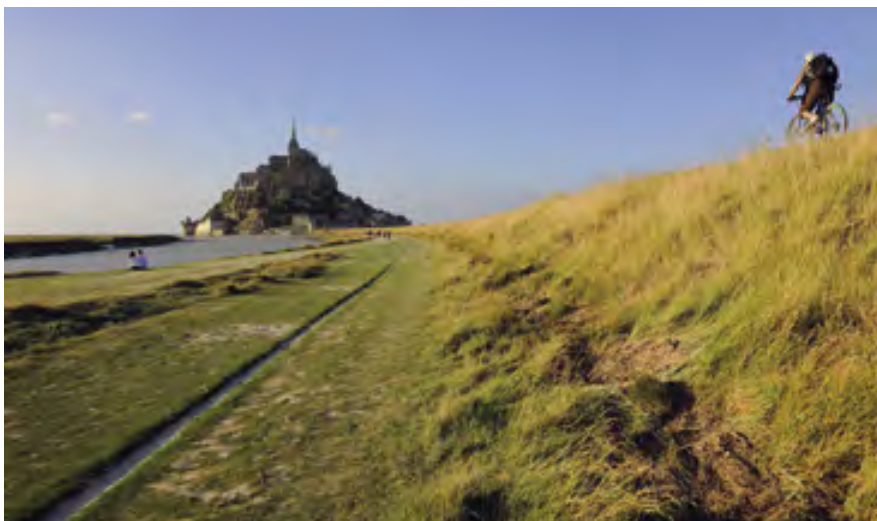
Source 3 This sea wall in Manche, France, is squeezing the salt marsh (centre) into a narrower strip as sea levels rise.
