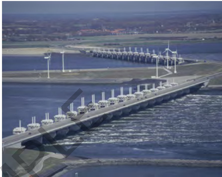
Source 1 The Oosterscheldekering storm surge barrier in Zeeland
