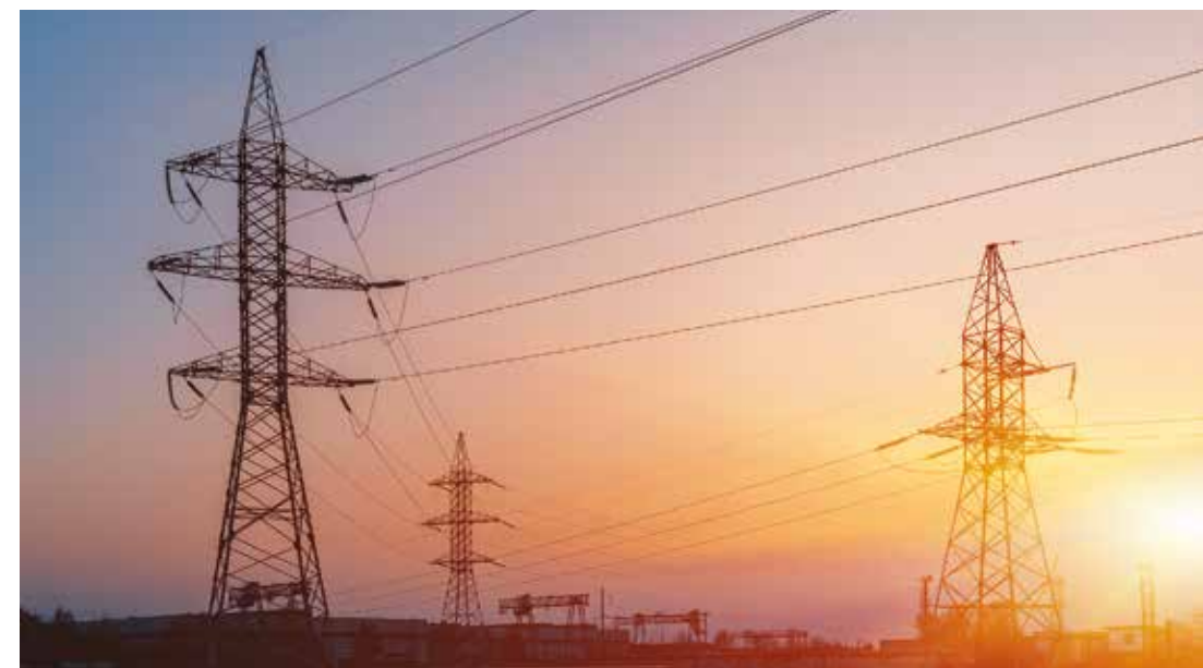
FIGURE 9 The magnetic field strength at ground level underneath these 500 kV power lines is over the 0.1 \mu\text{T} safe level. You have to be 150 m away for it to be safe.
