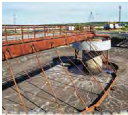
Figure 2.32 Flocculation results in the clumping together of suspended particles in waste water.
