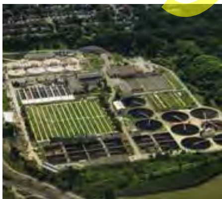
Figure 2.31 A water treatment plant.
